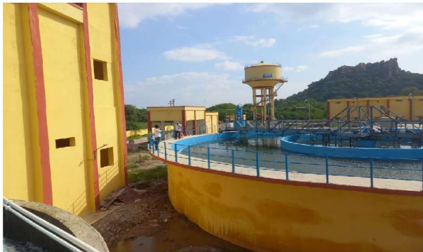
Water testing facility (Photo: Indal Kashyap)
